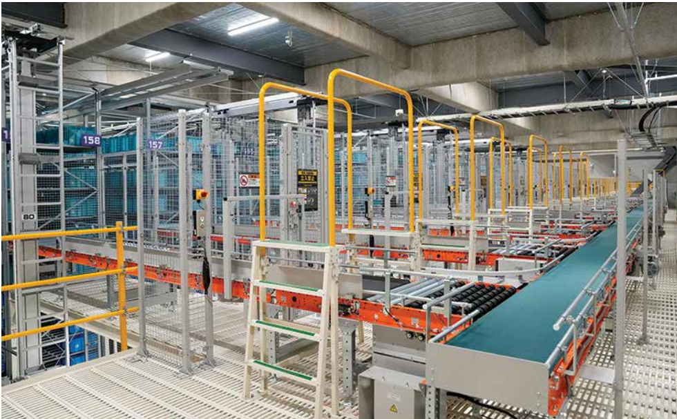
SB Logistics installed the conveyor and sortation system on a mezzanine level.
